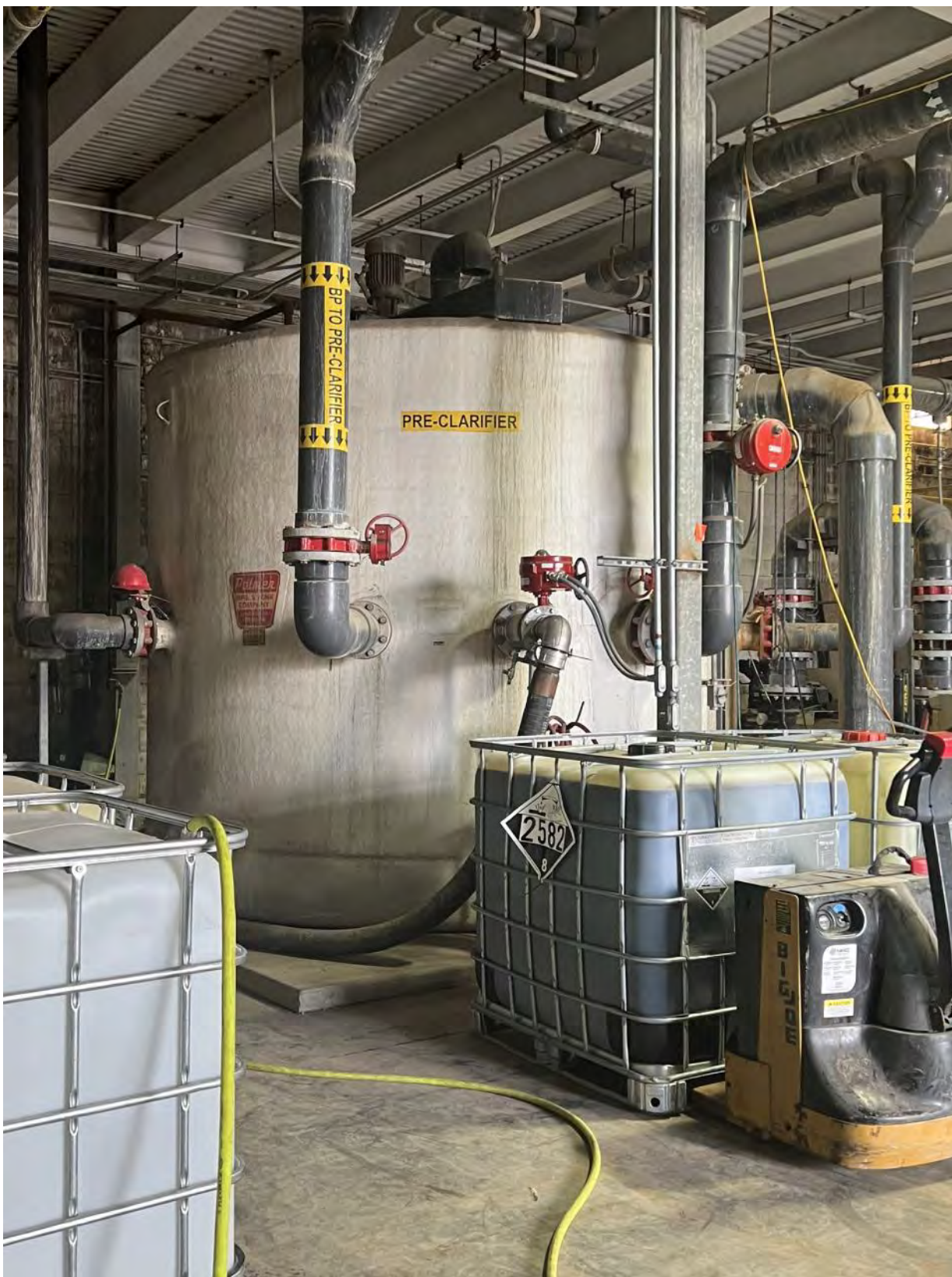
Pre-Clarified Filtrate Tank
