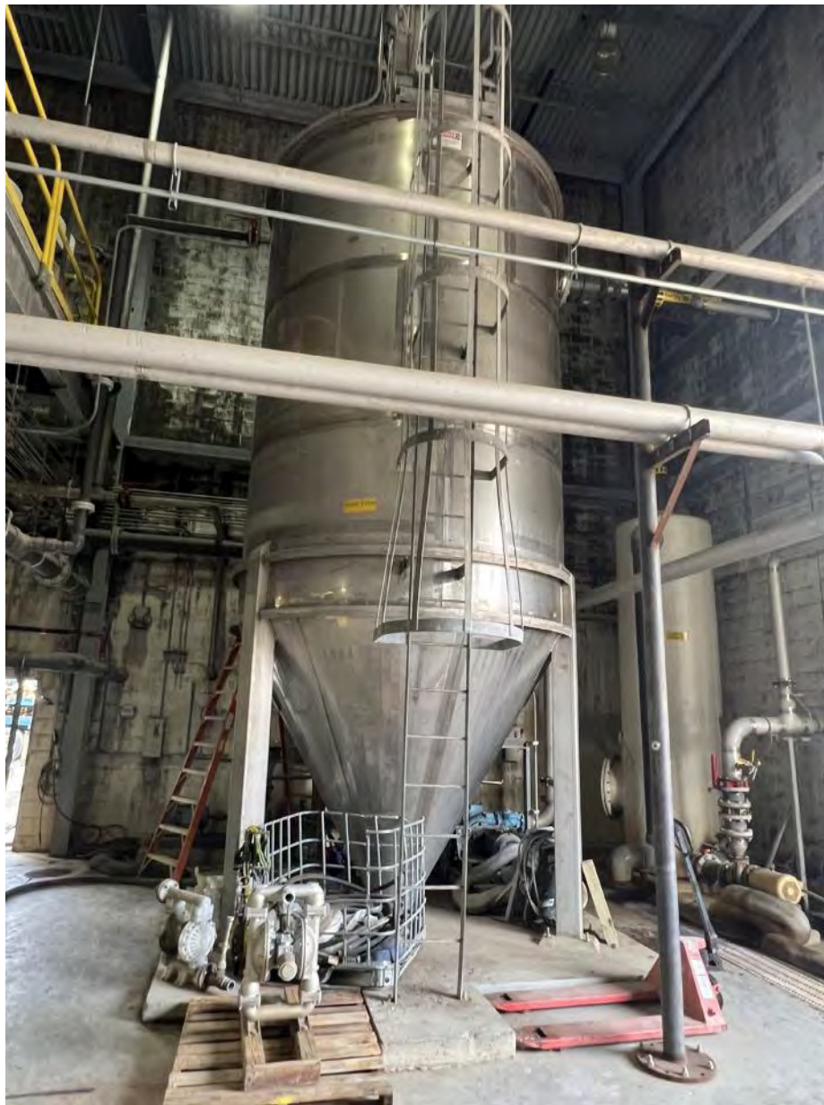
Continuous Blowdown Sand Filter
