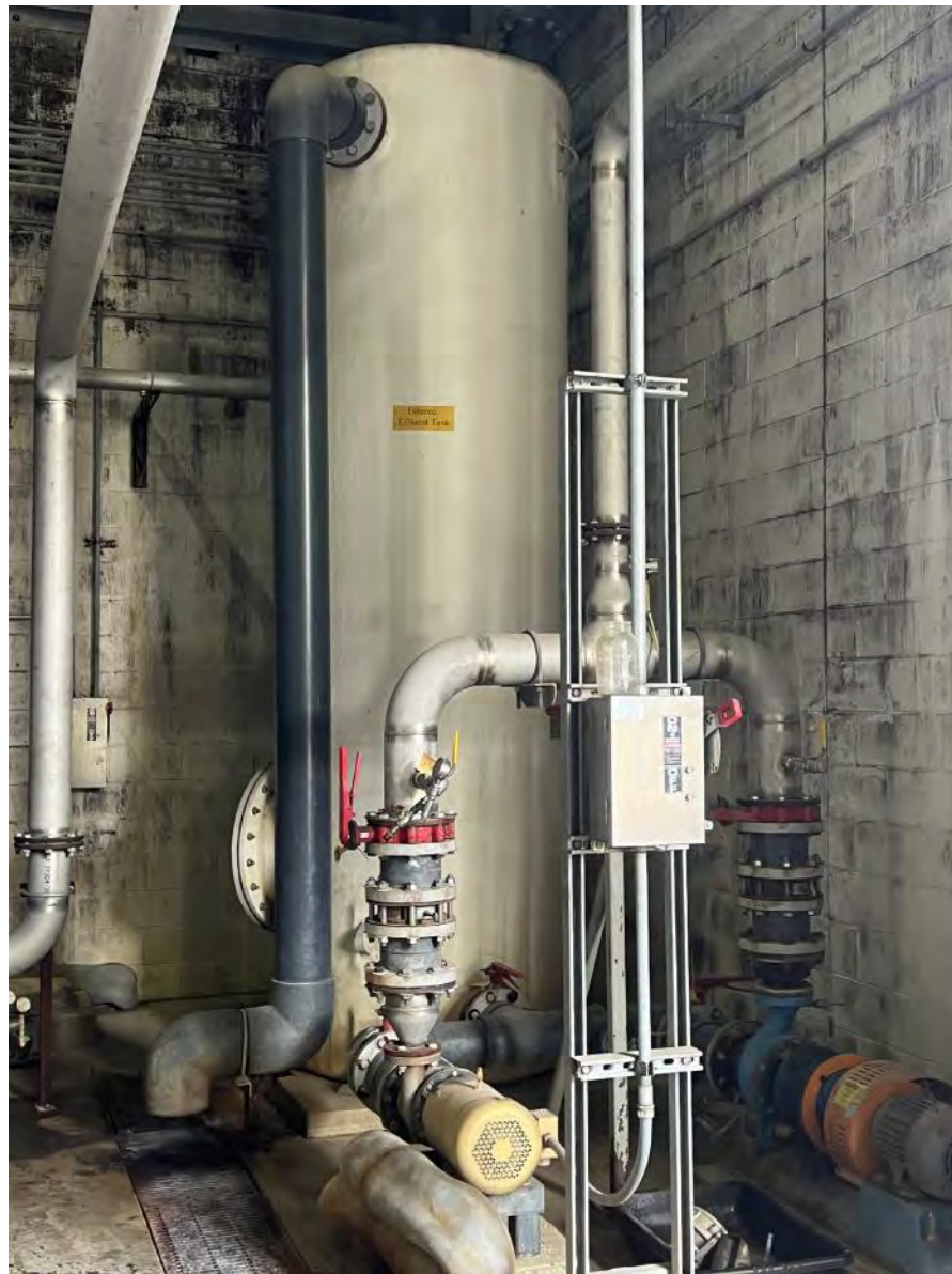
Filtered Effluent Tank
