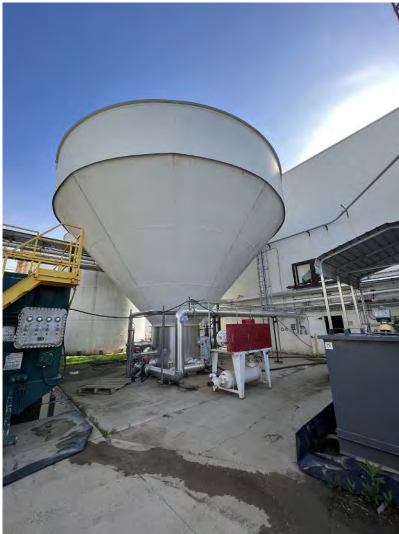
Solids Contact Clarifier (Original from AltEn System)
